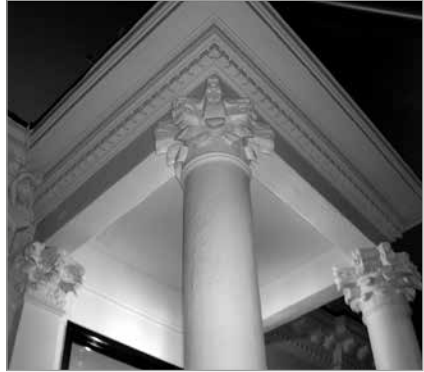
No 69 - recent repairs to the Corinthian capitals
